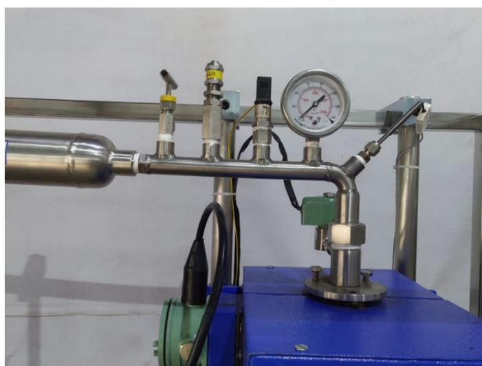
Figure 26: Manifold of the System
